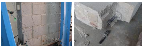
(c) Shear crack of masonry block and threaded rod broken
