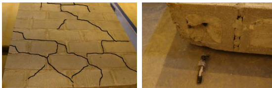
(b) Shear crack of masonry wall and threaded rod broken
