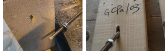
(e) Local crack of masonry block and bolt broken
