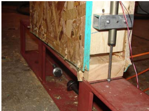
d) Separation of stud from bottom plate
