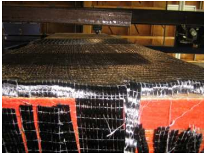
(a) Failure of FRP membrane in FRP-1
