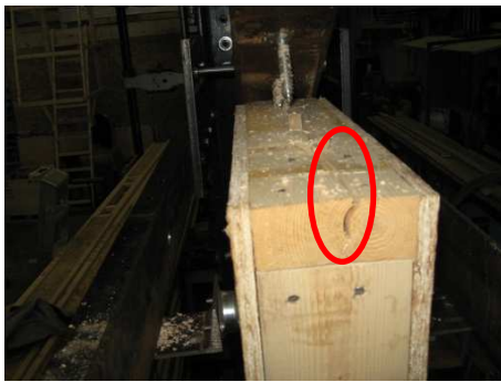
(b) Failure of bottom plate in FRP-2
