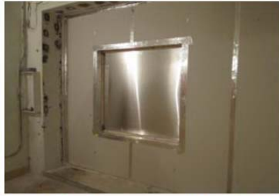
Figure 2 The test specimen installed in the filler wall
