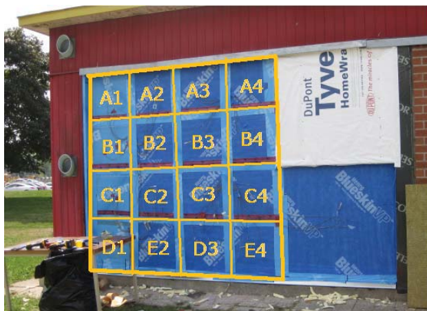
Fig. 6. After installation of water resistive barriers
